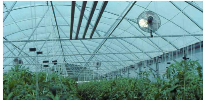
Figure 27. Horizontal air-flow fan for circulating air in greenhouse.
